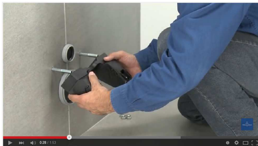
How to install - SupraFix 2.0 | Villeroy & Boch
